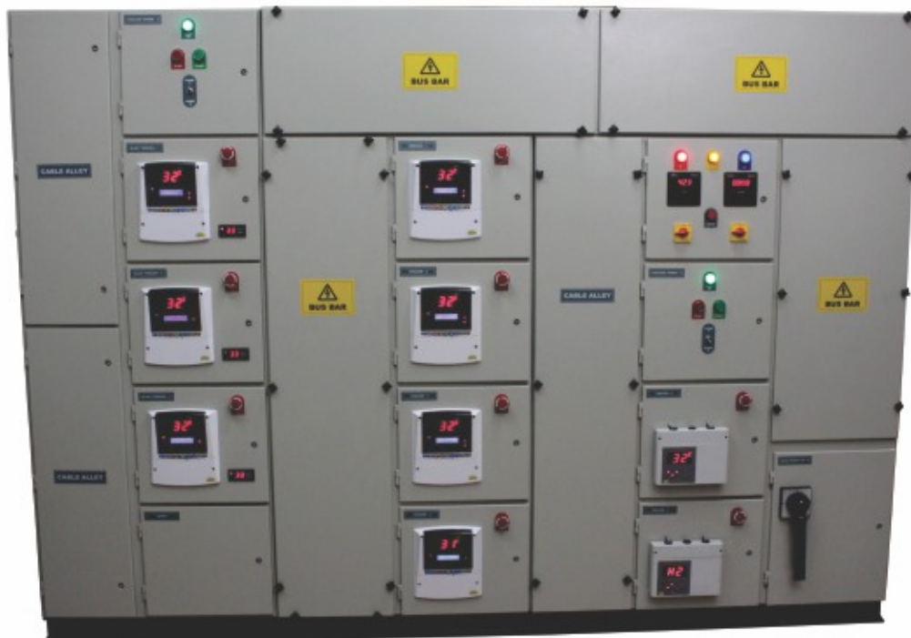
Multi Coldroom Electrical Panel
