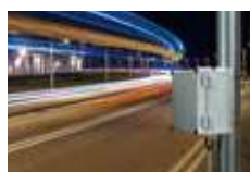
Pipe and post installation of enclosures
