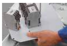
Device installation on mounting plates
