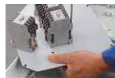
Device installation on mounting plates
