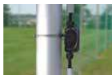
Pipe and post installation of enclosures
