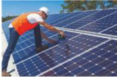
Requirements of the Solar industry
